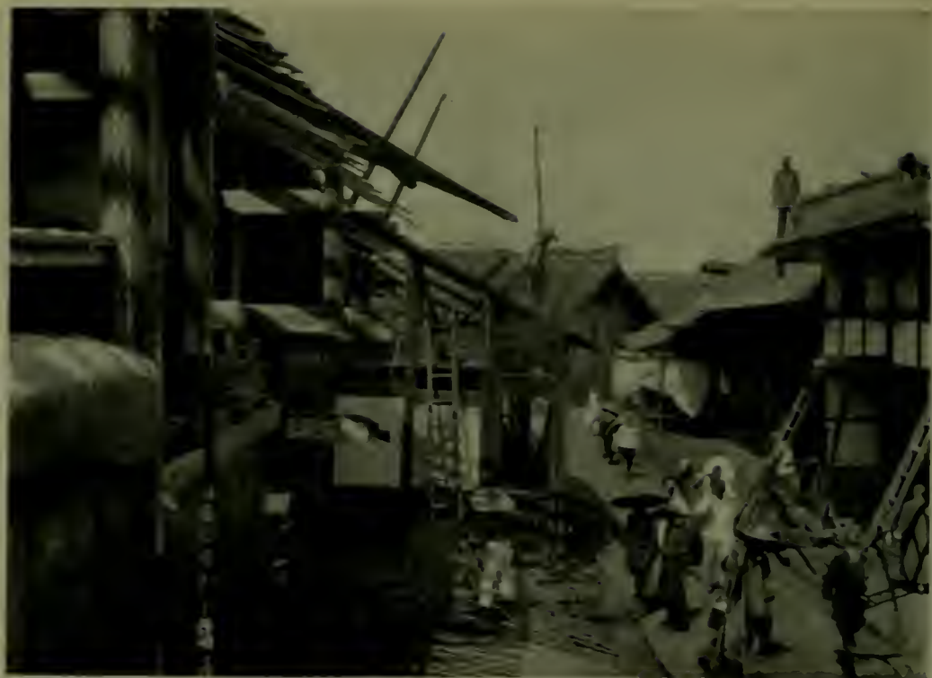
Under the ruthless orders for street-widening many a Chengtu shopkeeper had to cut away his whole shop in front of the dwelling occupying the back half of the building
